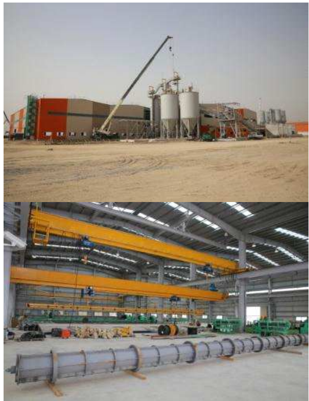
[PHC Pile Plant]
